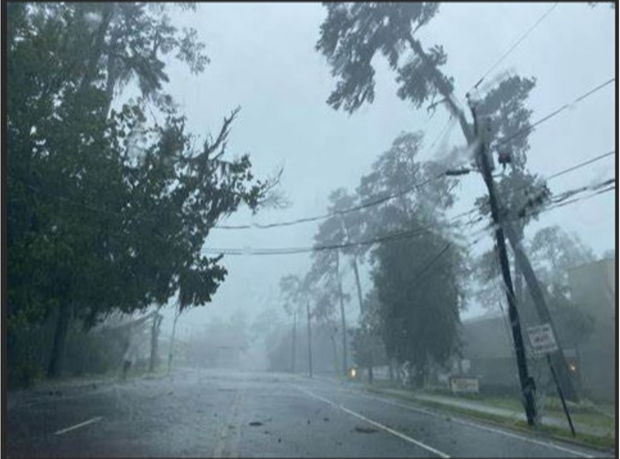
Photo: Idalia storm damage in South Georgia, 2023
