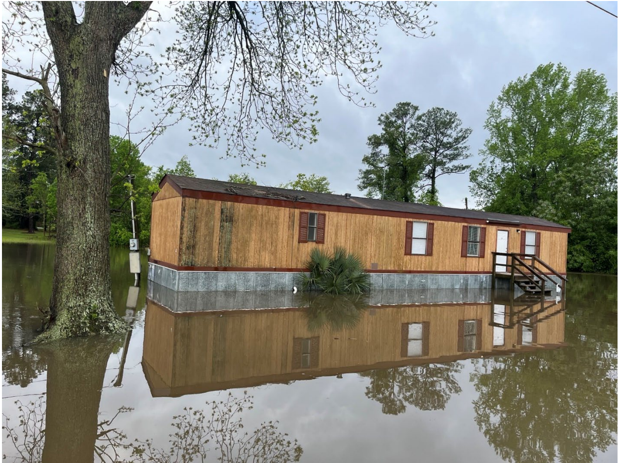
Flooding in Berrien County March 26, 2024
